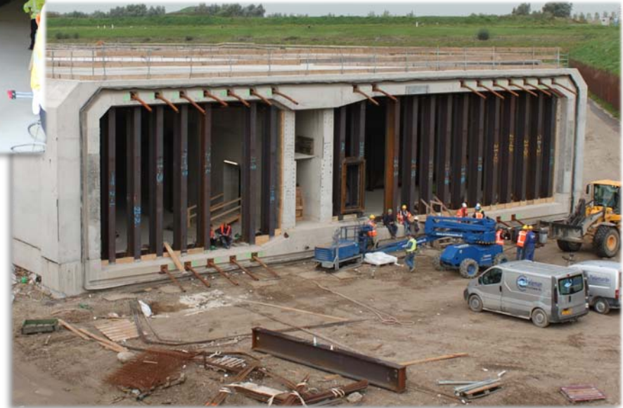
Adding end bulkheads
