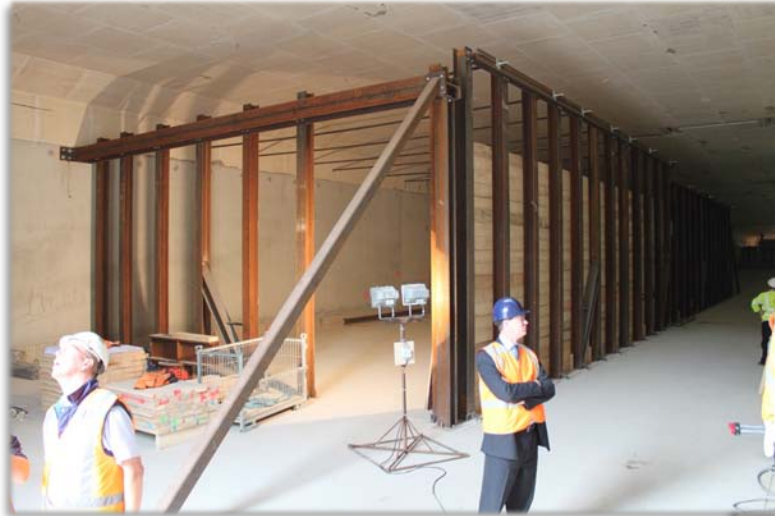
Ballasts tanks built into tunnel sections
