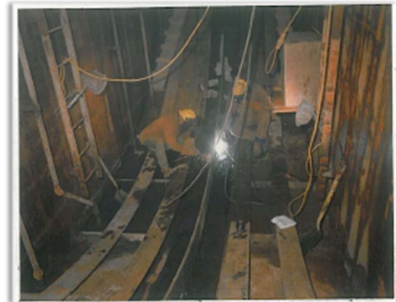
Making the connection between elements
