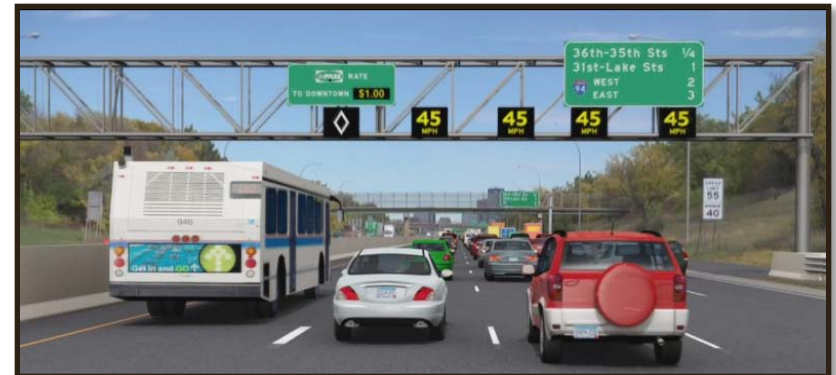
Managed Lanes (Part-Time HOV Lane, Hard Shoulder Running, Speed Harmonization, Queue Warning)
